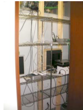
図7 玄関横の物入れの様子 Fig.7 A Storeroom by Entrance
